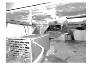
10. Hang the compressor assembly under the stove on the bolts. Tighten the bolts to secure.
