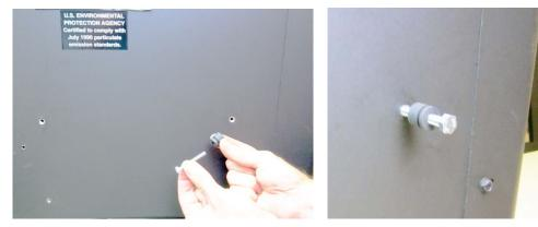
2. Tighten the bolts until the grommets contact the heat shield.
