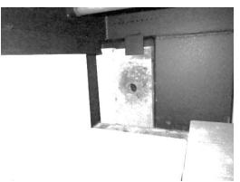
2. Remove the cover plate and 2 screws from the heat shield (located on the back of the stove). Retain the screws.
